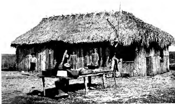
A trapper's home in the Everglades. The cabin is built of cypress bark and palmetto leaves
